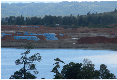
Figure 4.8: Reclamation in the Karkar area
