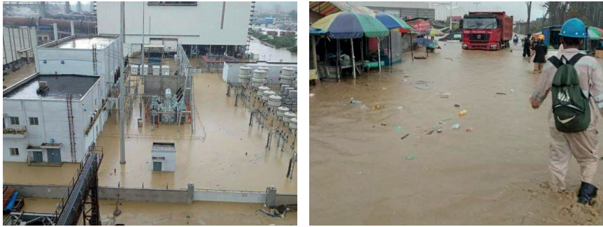
Figure 4.13: Floods inundating the IWIP area
